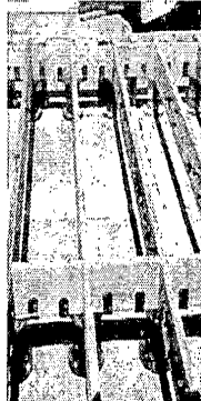
PEDESTAL SYSTEM WITH PAINTED 2X PT FRAMING AT WALKWAYS. GUARDRAILS TO BE ANCHORED TO 2X FRAMING. SEE PLAN FOR THE DOWN LOCATIONS AT DECK AND WALKWAY
